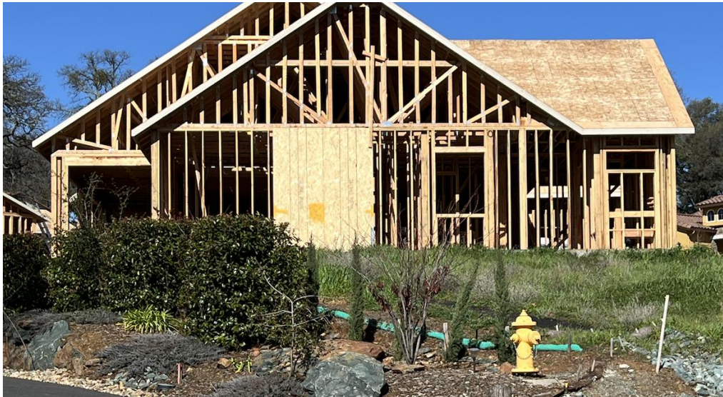
New home construction. (Photo: Katy Grimes for California Globe)
